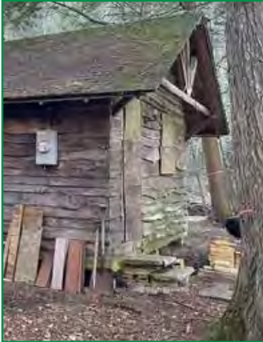
Nov. 12, 2023 – Cabin condition before repairs
